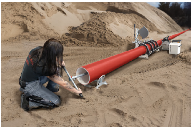
Cutting the welding bead using HÜRNER's Internal bead remover 300
